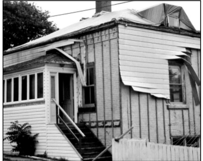
*The South West corner with wood strapping still showing painted brick. Some of these areas are unpainted under the porch roofline and this checkerboard is evident there. There is a starter course at the door threshold level which again projects one inch. Some brick has been damaged by strapping applied to hold the*
