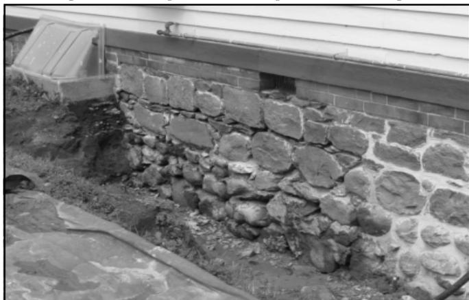
foundations. To the left is the cleaned area of foundation awaiting the parging which can be seen completed on the right hand side of the photo.
